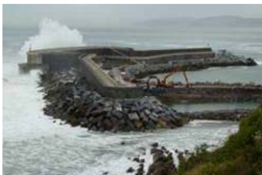
1) The Mutriku wave power plant in Northern Spain.*
