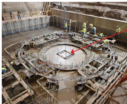
Pit during construction
